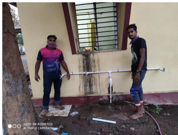
Wash Station built at the Saiwan Primary Health Center- Dahanu
