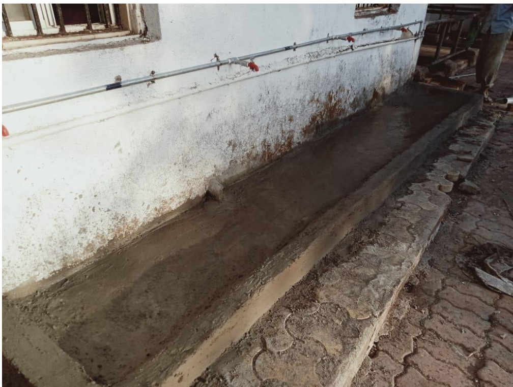
Wash station built at the Mokhada Rural Hospital
