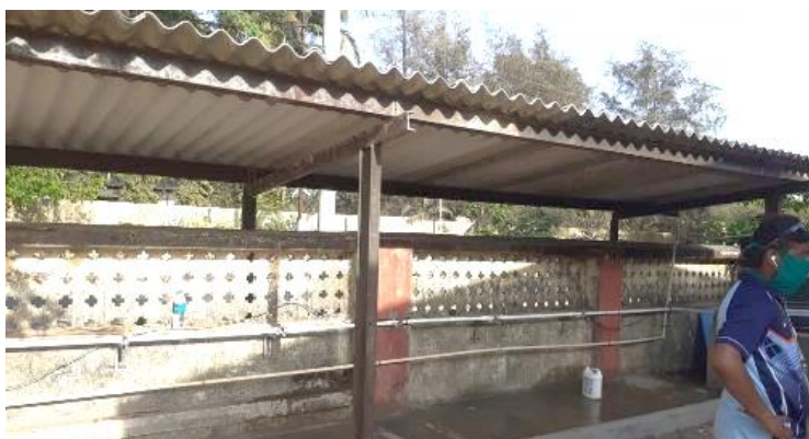
Wash Station built at the Dahanu District Hospital
